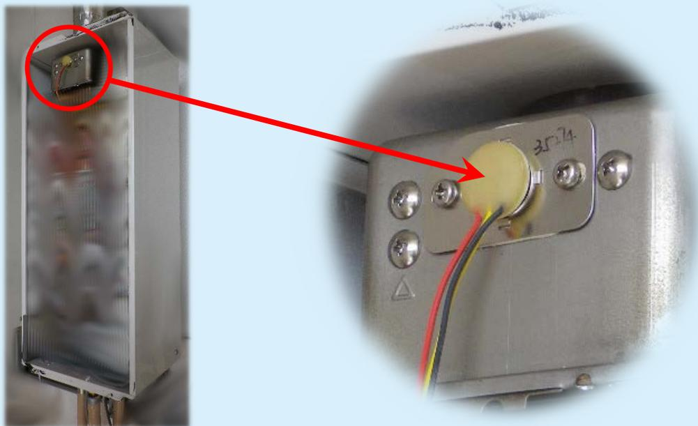
This arrangement will allow gas from the flue to diffuse to the sensor, allowing measurement to take place without interference from turbulent flows in the flue itself, and protecting the sensor from condensing conditions.
